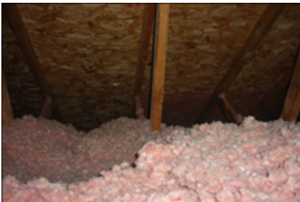
Over 15 inches of insulation
