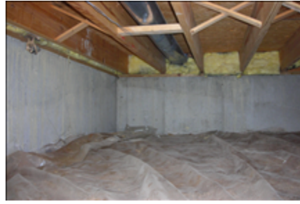
Insulate Floor and Duct in Crawl Space
