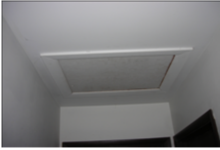
insulate and seal attic access
