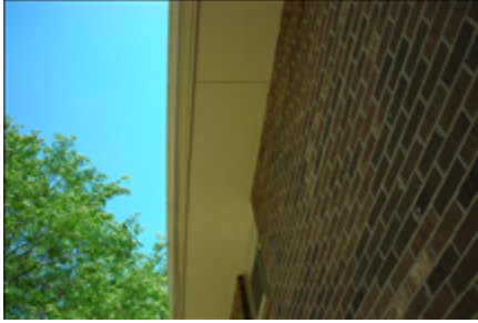
install attic intake vents
