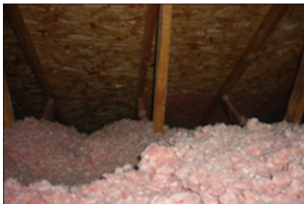
Over 15 inches of insulation
